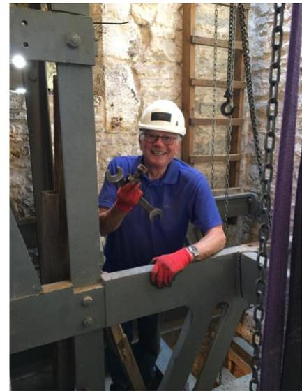
The third bell down was **Bell 3** and 1 and 2 were still tucked inside the raised frame. Three bells safely down by 11am. Time for a short coffee break. Now some of the frame had to be dismantled to get at **Bell 2** and **Treble**. Gordon managed to get out the first nut at 11:30 so the 2 bells were safely lowered to the ground by 1pm. By now the fears of working over the open trapdoor were abandoned as it was not as scary as had been imagined.
