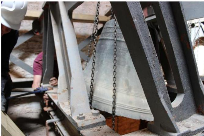
Andrew knew we were going to have a problem with the tenor as it was going to be too wide to pass through the frame where the fifth had hung. The headstock had to be removed but still no luck despite tipping it slightly and pushing it with some hefty boots! Nuts and bolts were removed from the frame but then they had
